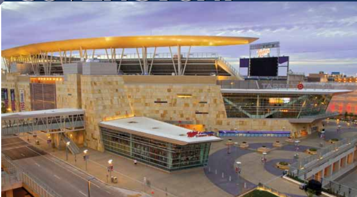
Target Field, home of the Minnesota Twins Major league baseball team has a champagne metallic canopy metal roof, which was painted on CSI's paint line in Columbia, SC. It is painted with a Versa Clad® 20 proprietary paint formulation of the Metal Dek Group®, a unit of Consolidated Steel Inc.
